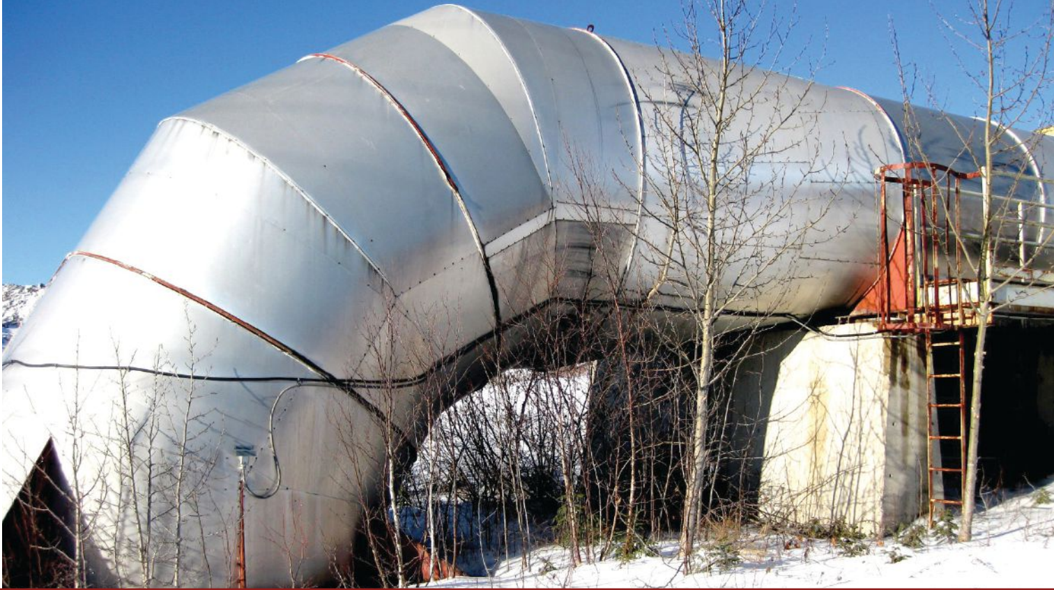
Ventilation is one of the largest contributors to carbon emissions in mining (along with diesel vehicles and ore processing). Photo: Stantec
