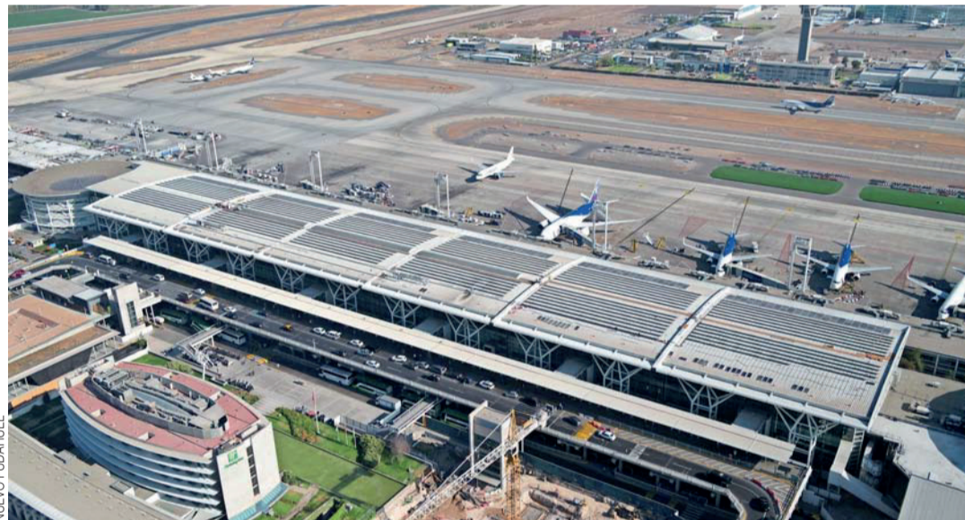
The photovoltaic plant installed on the roof of the old terminal (T1) consists of 2,465 modules that can generate 1,220 MWh/year.
